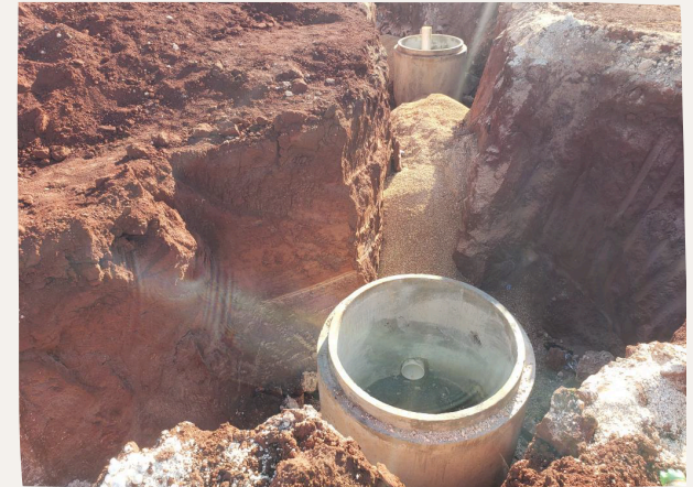
Sewer Manhole & Pipe Laying
