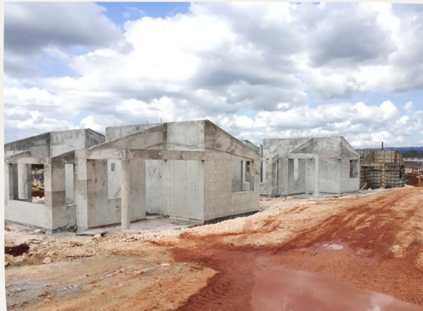
Concrete Walls after Pouring
