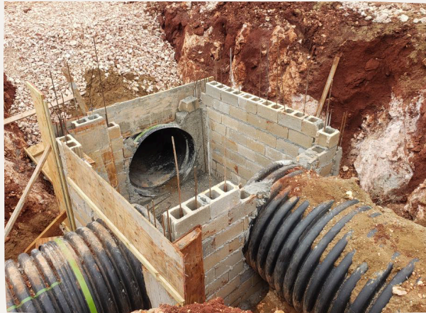
Inlet Stormwater Erection
