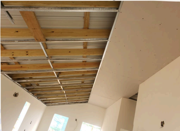
Drywall Ceiling Installation
