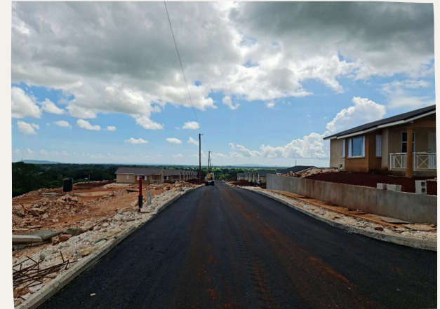
Asphalt Road Paving
