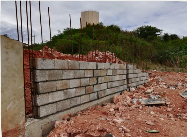
Retaining Wall Erection
